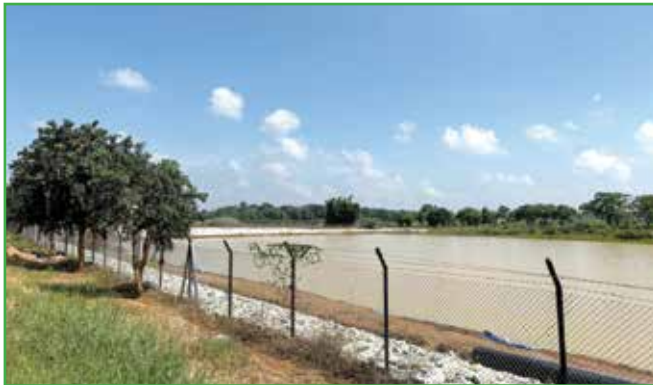
Rain water harvesting pond
