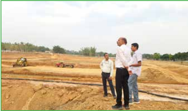
Farm pond digging
