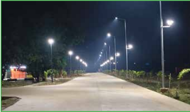
Internal roads along with street lights
