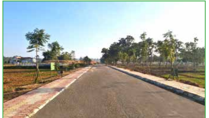
Paver block laying and avenue plantation
